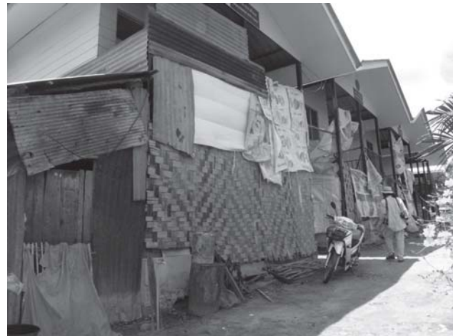
Figure 3: The mismatch between the architectural characteristic and dwellers' living space
