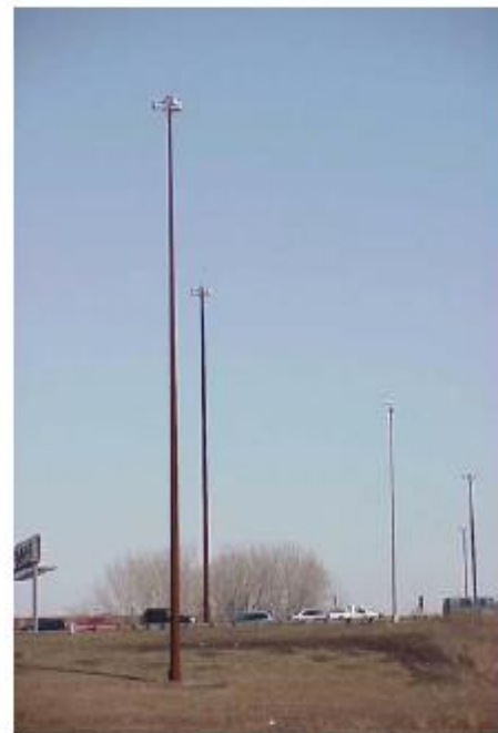
High Mast Tower Poles (3-100, 4-100, etc.)
