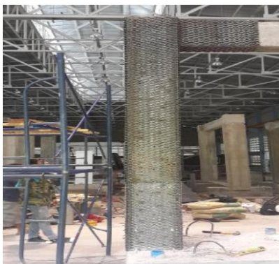
(a) Strengthened bare frame with expanded metal
